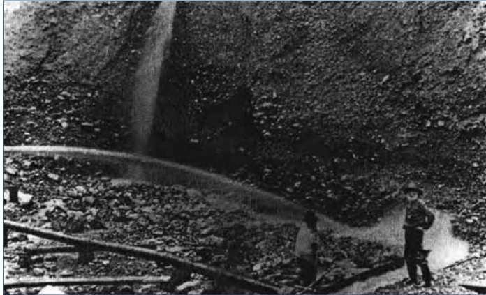
Fig. 5b. Hydraulicking lodgement till and underlying gravels on the upper part of Lowhee Creek, 1930's.
