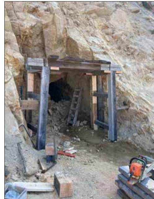
(above) Collar construction. (below) Collar completed.
