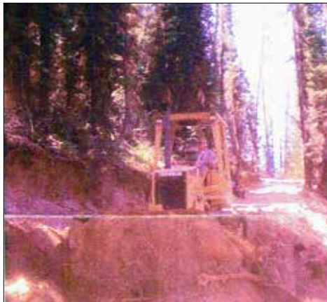
Bill Brown building road access.
