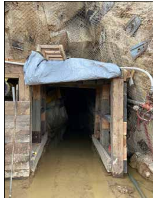
(above) Collar construction. (below) Collar completed.
