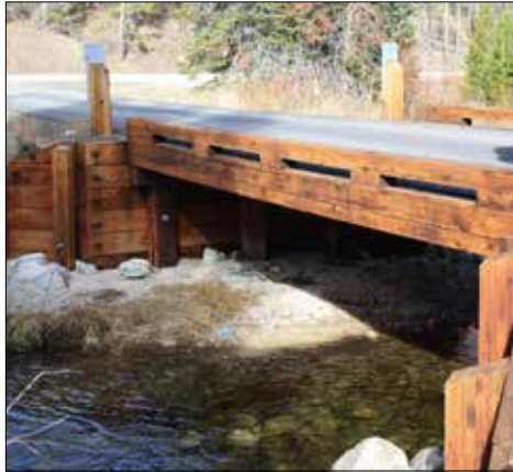
Bridge over Steamboat Creek.
