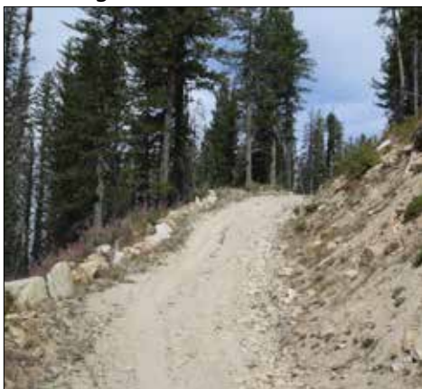
Road access, Nov. 2012.
