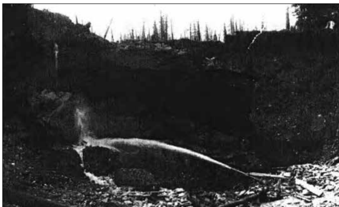
Fig. 6b. A face being hydraulicked at Stouts Gulch. Note large blocks of lodgement till fallen from face.
